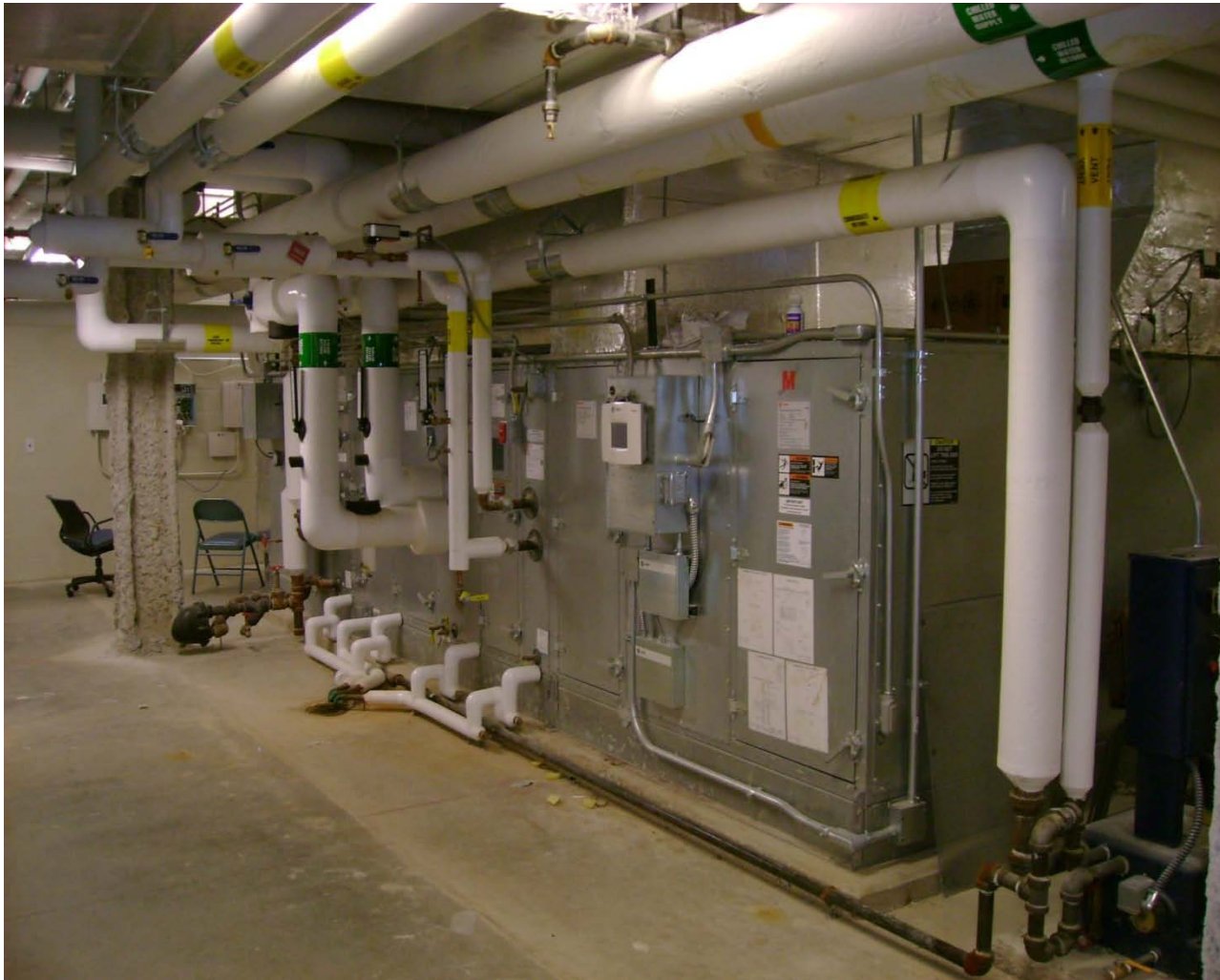
Typical Air Handling Unit Chilled Water Coil- 42 degree F water Hot Water Coil- 150 degree F water
