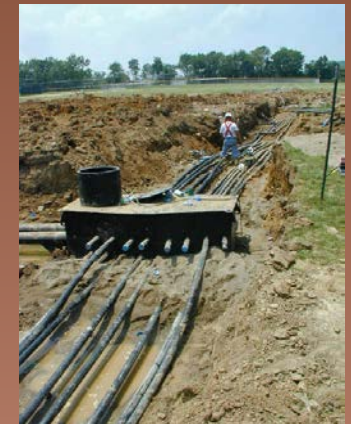
Commercial ground-coupled (closed loop) heat pump system
